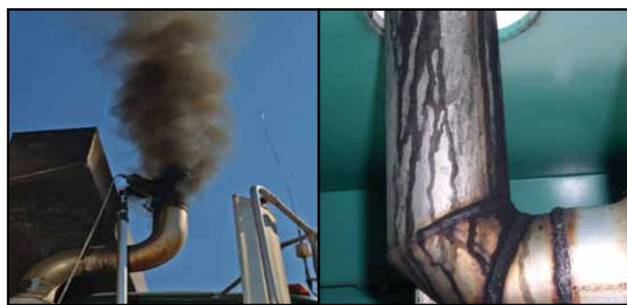
“The Accumulation of Unburned Fuel or Carbon on a Diesel Generator’s Exhaust Side”
