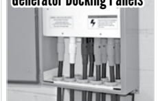
Generator Docking Panels
